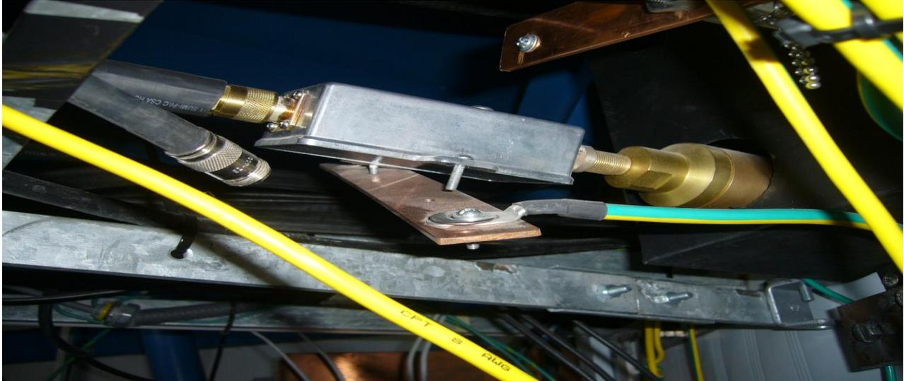
9. Coaxial Cable Signal Lines Showing Improper Installation
