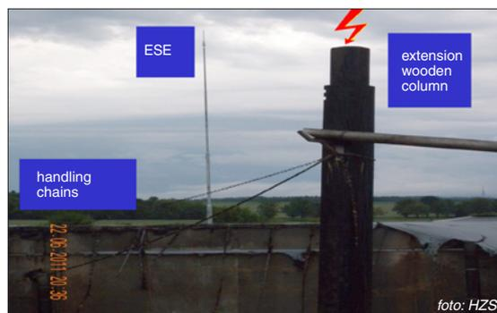
Fig. 3. The damaged technological part of fermenter after lightning strike in a protective area ESE
