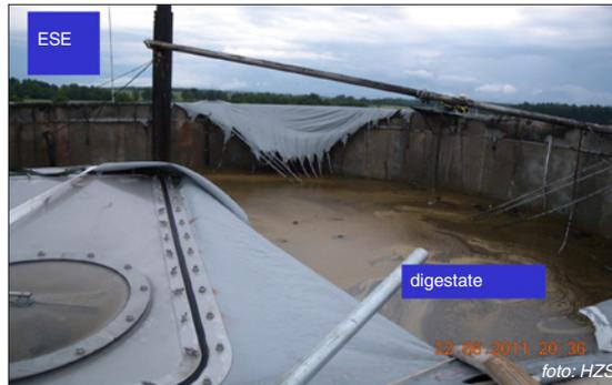
Fig. 6. View into the damaged inner tank of fermenter, which is located in the protective area of ESE
